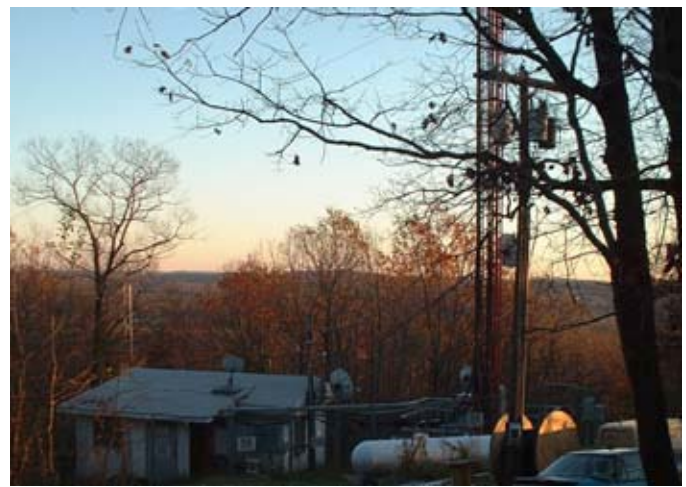
Wintry sunset at the 2m/440 repeater site. Because of problems with the Diamond dual-band antenna on the tower, Bob N2CBH has transferred the PCARA 2 meter repeater back to the Sinclair twin folded dipole antenna just visible above the roof.
