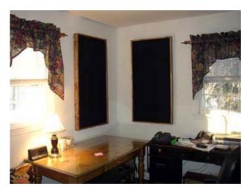
WB2HNA's new radio room is quiet as a mouse thanks to six sound absorption panels covered in black speaker cloth.
