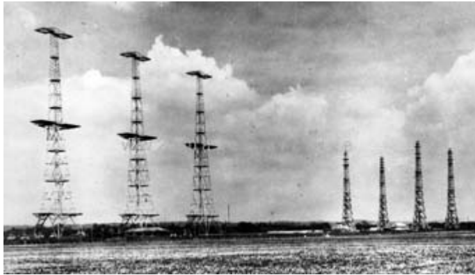
Chain Home radar station at Poling Sussex, with three 350 ft steel towers for transmit antennas and four 240 ft wooden towers for receive antennas. [RAF photo.]
