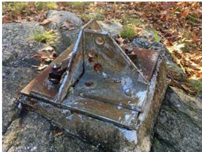
*This hardware likely held guy wires for the Bilby Tower, which was located about 20 yards away. The W2IGG antenna mast was affixed to this bracket. [KD2ITZ pic.]*
