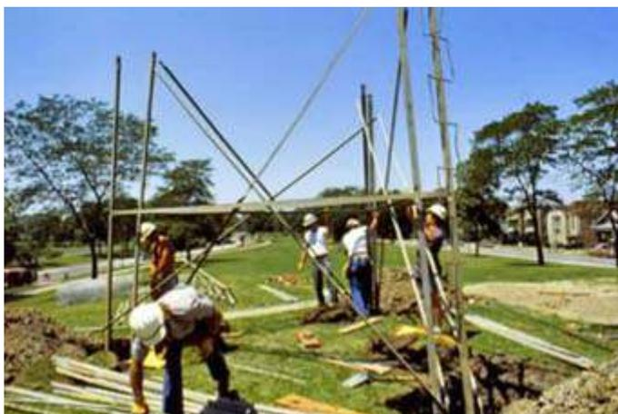
Construction of Bilby Steel Tower. First sections of the inner and outer tower have been built, to a height of 13' 8".
