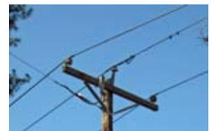
*Utility pole carrying three high voltage wires for three phase primary.*
