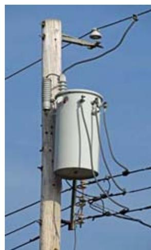
*Pole-mounted transformer steps down the 13 kV primary to 120-0-120 volt, center tapped, for distribution to nearby homes.*
