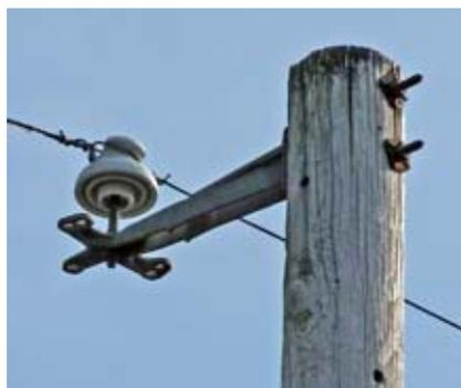
*Porcelain "pin" insulator on utility pole supports 13 kV primary conductor. Extended surface under insulator stays dry in rain and snow.*
