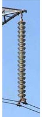
*High voltage insulator for 275 kV line.*
