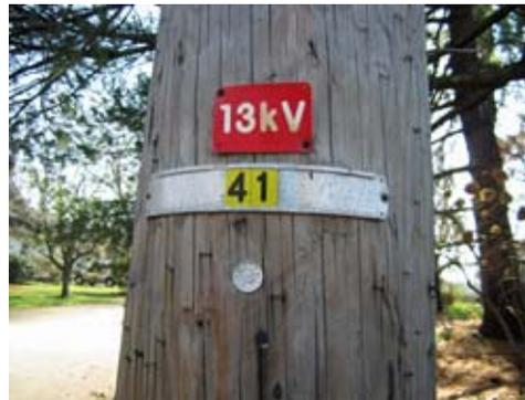
*This ConEdison utility pole is clearly marked with the primary voltage.*
