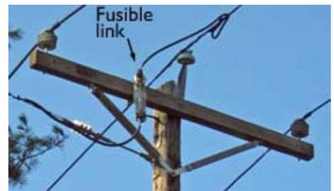
*Fusible link on 13kV primary will hang down when fuse has blown.*
