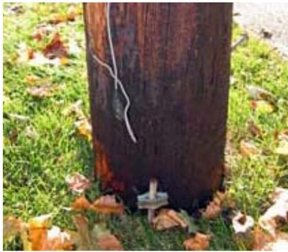
*Broken ground wire at the foot of a utility pole.*
