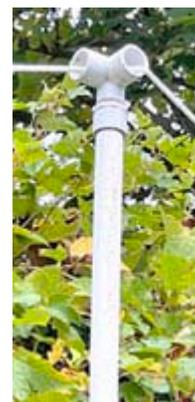
PVC pipe and 90° 3-way elbow guides the support rope.
