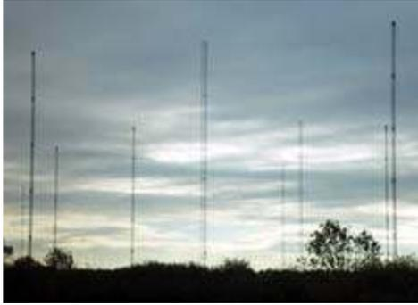
*Twelve 820 ft masts supported the 16 kHz wire antenna at former VLF transmitting station GBR, Rugby.*
