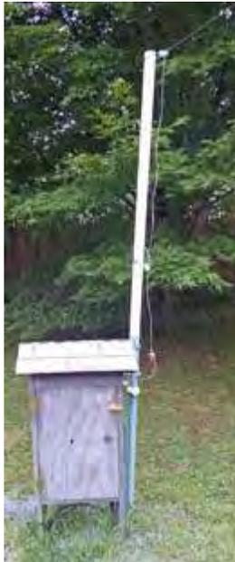
Antenna tuning unit is enclosed in a wooden shelter. [N2CBH pic]
