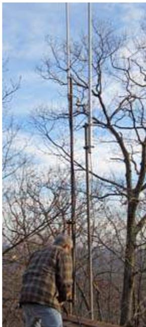
Antennas at the repeater site. The Diamond dual-bander for 440 MHz is on the left-hand mast.
