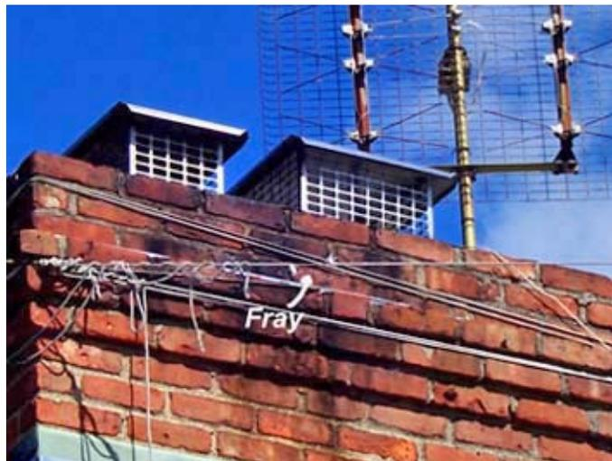
*It's the time of year to check your antennas and supports. Here is a recently-discovered frayed rope, barely clinging on to Karl's chimney.*
