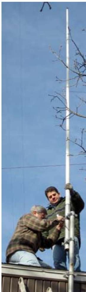
Bob N2CBH and Rich WZ2P install a VHF gain antenna at the W2NYW repeater site in 2012.
