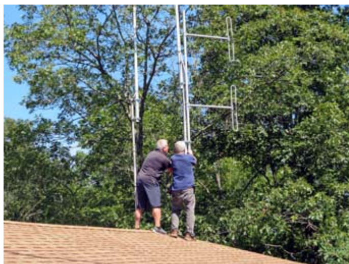
Rich WZ2P and Bob N2CBH install the Sinclair 2-bay exposed dipole antenna.
