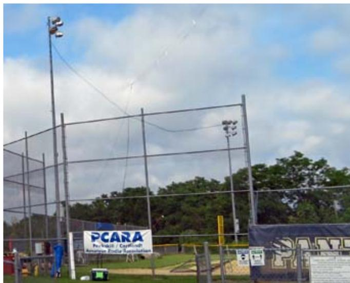
View of east and west light poles, supporting catenary rope for wire beam. (Catenary and feeder are emphasized.)
