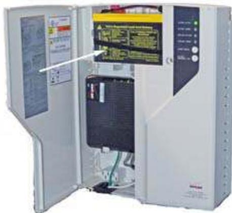
Verizon Fios box contains a sealed lead acid battery (arrowed) for battery back-up in the event of a 120V AC power failure.
