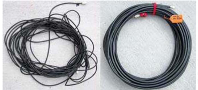
Don't store your coaxial cables in a tangled mess. Roll up neatly and use Velcro cable ties to keep the turns together.
