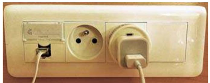
French power outlet has ground connection pointing outward.
