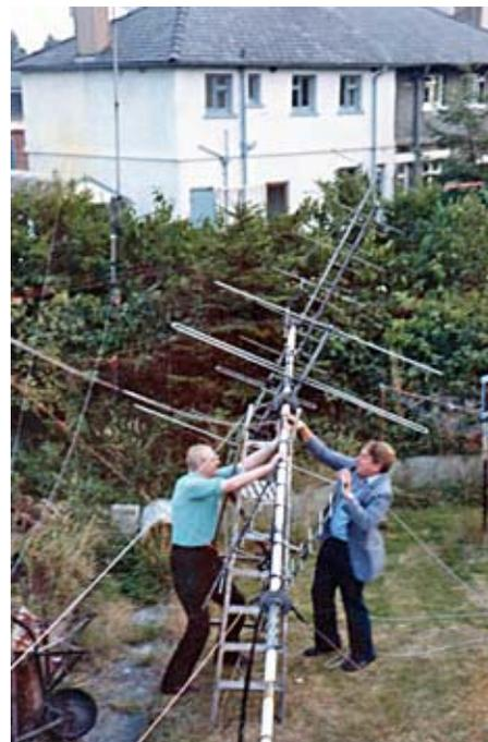
*Work on the VHF antennas at G3VNQ, Southport, with Wilf, G3STT (left) and Harold, G3LWK assisting. The 4 meter 3 element yagi is lowest on the mast.*
