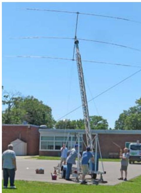
*Raising of the three-element tri-band beam on the tilt-over tower.*
