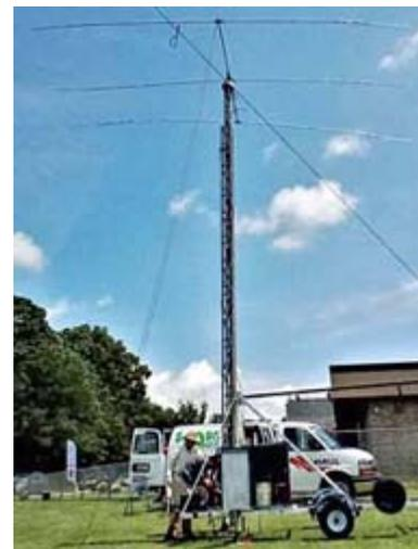
*Tri-band beam on the tower. [Ray K2RCQ pic.]*
