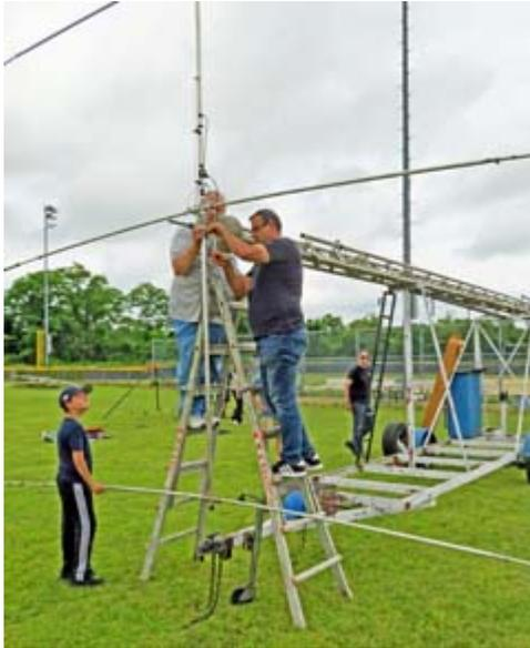
Joe's renovated TH3Jr tri-band beam is attached to the mobile tower.
