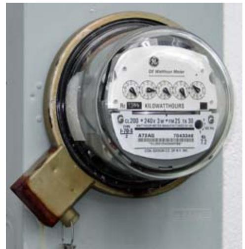
*Electricity meter outside the home indicates a steady current draw with nothing switched on.*
