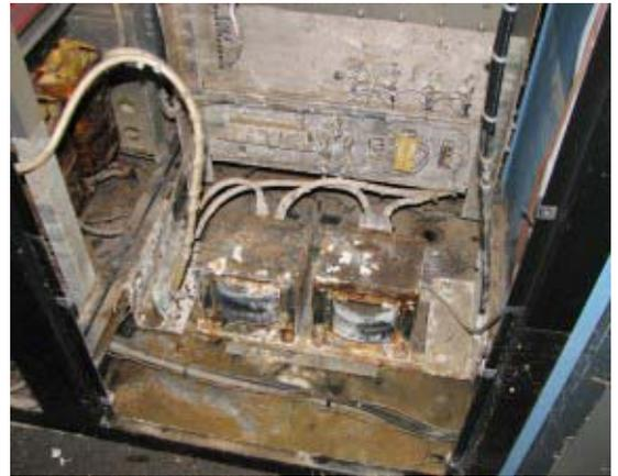
*WMCA's Nautel transmitter was flooded in 2 feet of water.*
