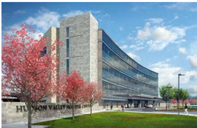
New patient tower at Hudson Valley Hospital Center
