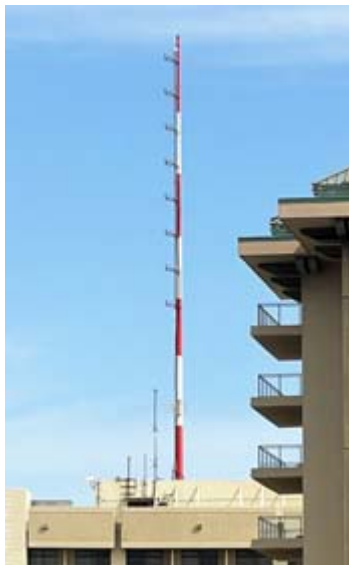
Tower for KHCM-FM has an 8-bay antenna stack.
