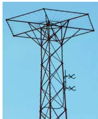
KHVH AM transmit tower with two-bay FM antenna under the capacitance hat.
