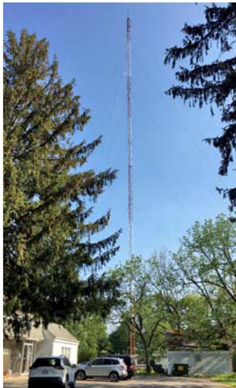
Grounded tower at WFAS is 450 ft high. It is surrounded by a wire skirt, fed at the base, constituting a folded unipole for MF transmissions. [N2KZ pics].
