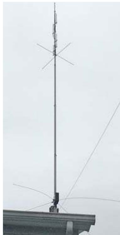
*Main antenna is a Cushcraft R5 vertical, seen here along with the 50 ft horizontal long wire fixed to the sewer vent pipe. [N2MUZ pic]*
