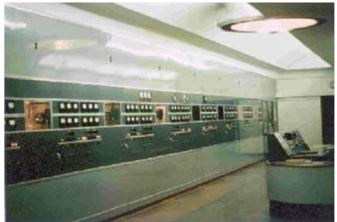
Aspidistra's underground RCA transmitter included three 170 kW PA units that were combined to produce 500 kW. When over-run they could generate 600 kW, which was fed to a three-mast MF array above the transmitter hall.
