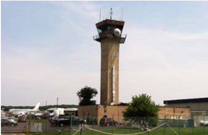
Control tower at Westchester County Airport, KHPN.
