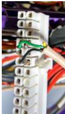
Wires for the ‘Power-on’ switch were simply pushed into the 24-pin connector.
