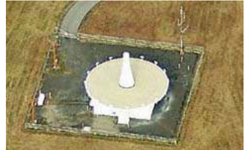
CMK ATIS and VOR/DME transmitter site near Rt 35 in South Salem.
