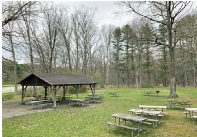
Picnic Shelter 3B near Parking Lot 3 in FDR State Park.
