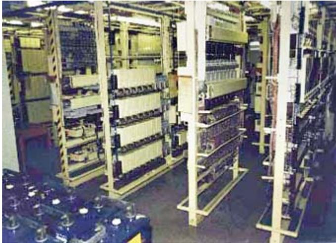
*Strowger equipment still in use at a British Telecom exchange in 1995. Lead acid battery at bottom left.*
