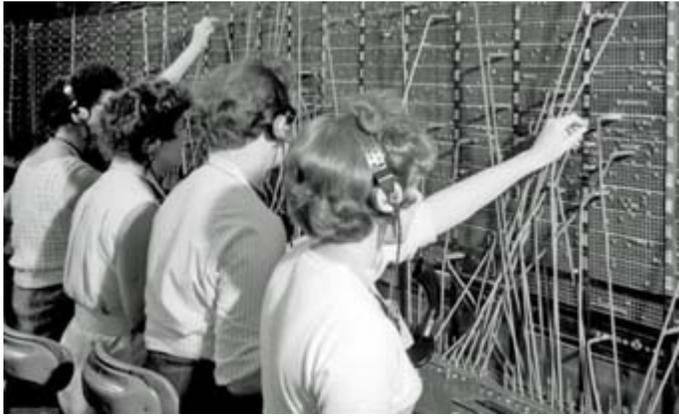
*“Number please?” A British telephone exchange of 1960 with female operators still connecting calls by plugging a cord into the outgoing circuit and ringing the recipient’s bell by pressing a key.*
