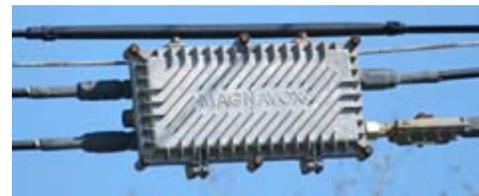
*Coaxial cable line extender hangs below a newer fiber optic cable.*
