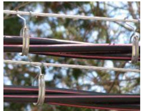
*Newer style shielded 13kV distribution cables are suspended from stranded steel messenger lines using cable rings.*
