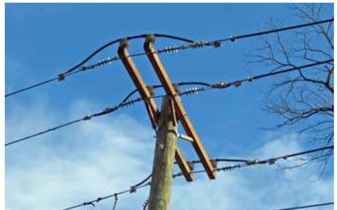
*The old and the new. Utility pole near Crompond Plaza carries older, thin wires with deteriorated covering to the left and new-style, heavy duty primary wires to the right.*
