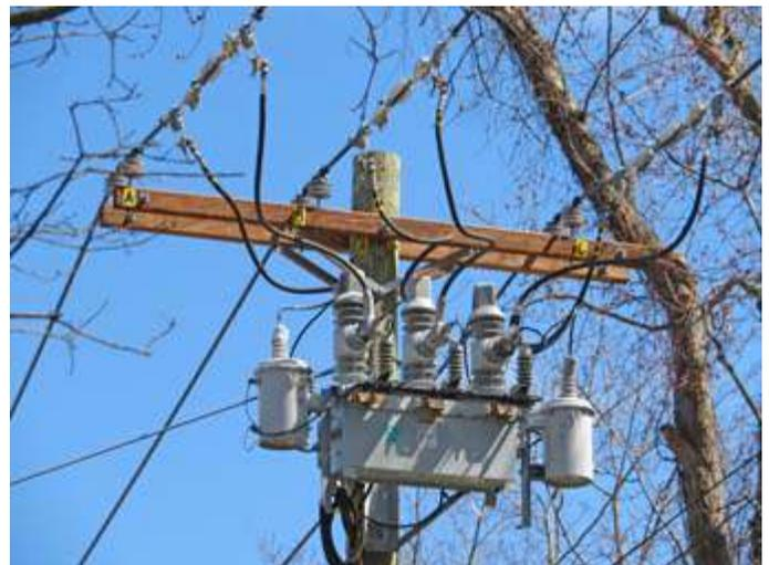
Con Edison “smart switch” or Kyle Recloser is installed on a newer pole at Route 202 and Dimond Ave. The switch can isolate sections of 4 kV feeder under remote control.
