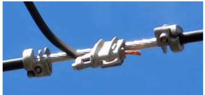
*Insulated copper tap wire for side street is clamped onto one of the new primary phase conductors on Rt. 202.*
