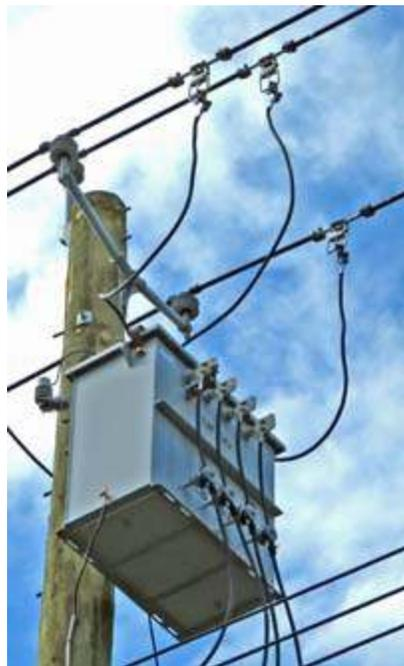
*Rectangular-shaped pole transformer supplies three-phase 208 V AC to commercial premises along Route 202.*
