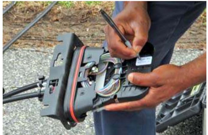
3M fiber closure being labeled prior to installation high in the air. Unspliced fiber strands are looped around the inside of the closure before they continue down the street.
