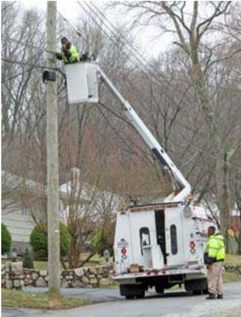
Two Optimum contractors make a loop of fiber-optic cable available at ground level alongside selected utility poles.
