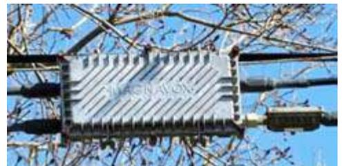
Bidirectional amplifier powered from coaxial cable extends the cable's range.
