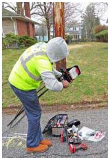
Cable loop is split open and inserted into a plastic closure.
