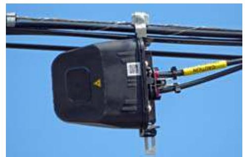
3M BPEO closure suspended high in the air on cable company steel wire. Yellow sleeve identifies Altice fiber optic cable.
