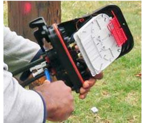
Close-up of 3M BPEO fiber closure with two splice trays inside, ready for connecting drop cables to the premises.
