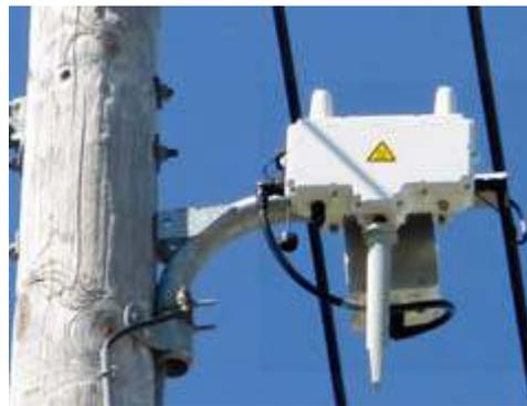
Close-up of access point. 902 MHz mesh antenna below, WAN/cell antennas on top.
