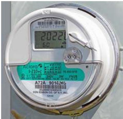
*Aclara I210+c Electric Utility Watt-hour meter. Meter form is marked '3W FM2S' (three wire service, 240 volt single phase).*
