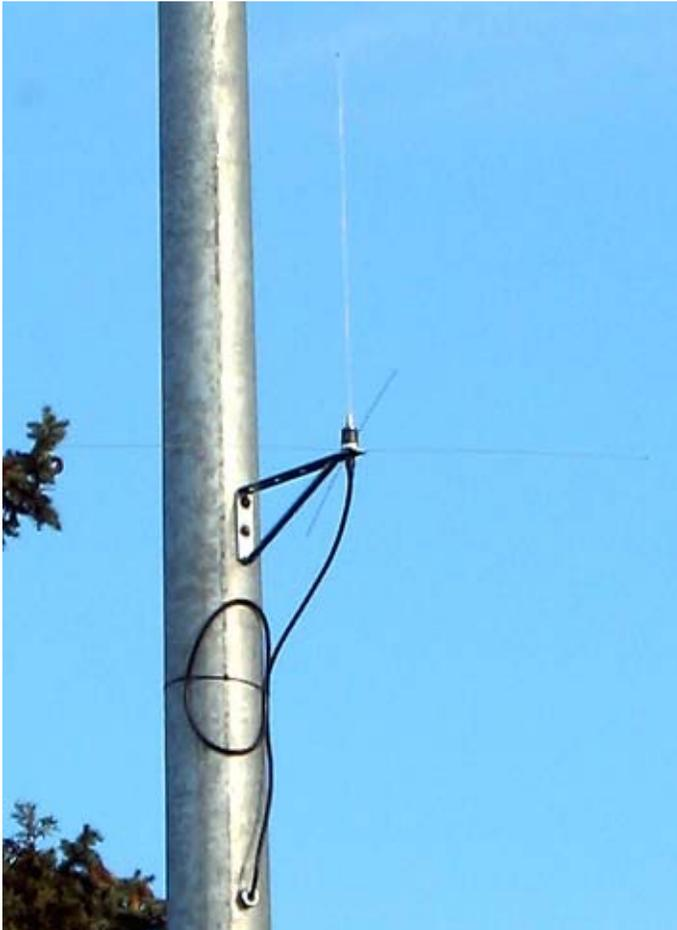
*Ground plane antenna mounted close to metal pole that supports the new stationary sirens.*
