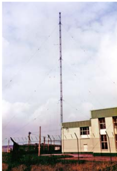
BBC Moorside Edge transmitter site in 1982. Twin 500 ft masts act as radiators and support wire cage antennas. [G3VNO pics.]
