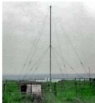
Decca Hi-Fix transmit antenna had a vertical mast with capacity hat consisting of the top set of guy-wires.
