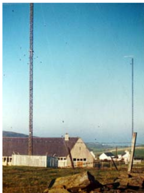
MF transmit antennas at Anglesey Radio pictured during a visit in 1977. Separate receive antennas were sited ~1 km away, fed with pressurized coax. [G3VNQ pics.]
