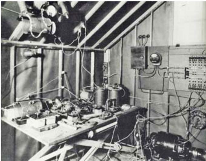
Transmitting equipment in the hut at 1BCG, Greenwich. Antenna coupling transformer is visible top left, four tubes lie horizontal on table and motor generator is bottom right.
