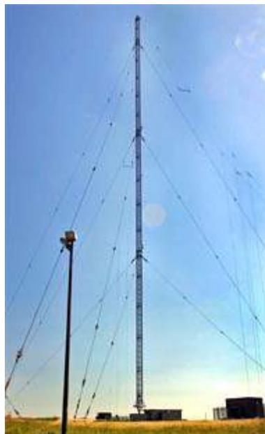
*Moorside Edge transmitting site in northwest England radiates three services including talkSPORT on 1089 kHz with 400 kW.*
