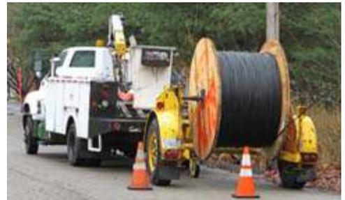
Prismian fiber optic cable was being unreeled down the length of this Cortlandt street, supported high on the utility poles.
