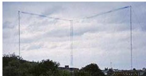
Two-wire "T" antenna suspended between guyed masts at a BBC MF site.
