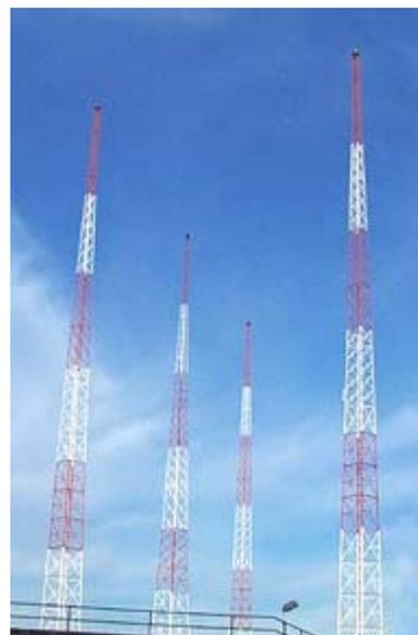
The four towers of WFME-AM, Maspeth, Queens. Two towers were used for the daytime pattern, three towers for the more directional night-time pattern.
