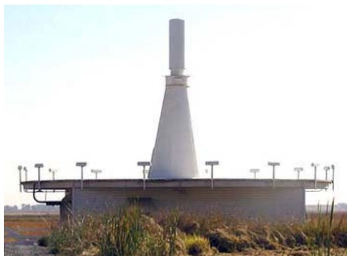
*VOR/DME characterized by a circular array of VHF antennas above a ground plane, plus a white, cylindrical radome housing the distance measuring antenna for 960-1215 MHz.*
