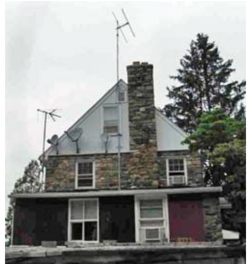
WJZZ transmit site near Brewster, NY. Slant-polarized CA-2FM antenna is visible above the chimney.
