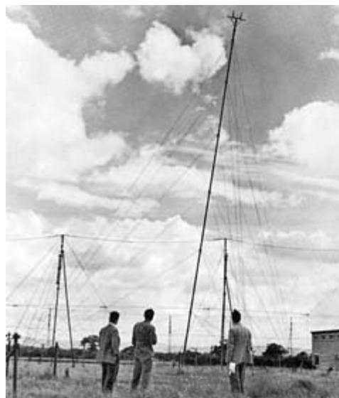
218 foot diameter wire paraboloid was fixed to the ground, with 126 ft mast carrying the antenna at the focus. Robert Hanbury Brown (center) would tilt the vertical mast to shift the beam slightly.
