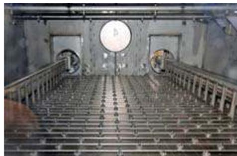
*Connections to the electrostatic precipitator rods at RSR, Wallkill.*
